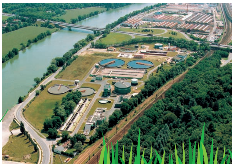
Credit photo CA Evry Centre Essonne - SEE
